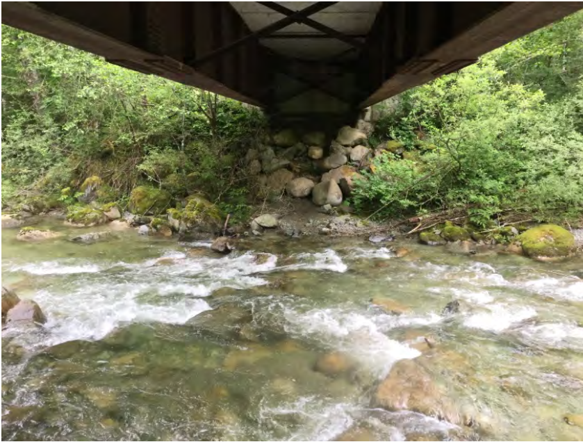
Right Bank Abutment when facing downstream
