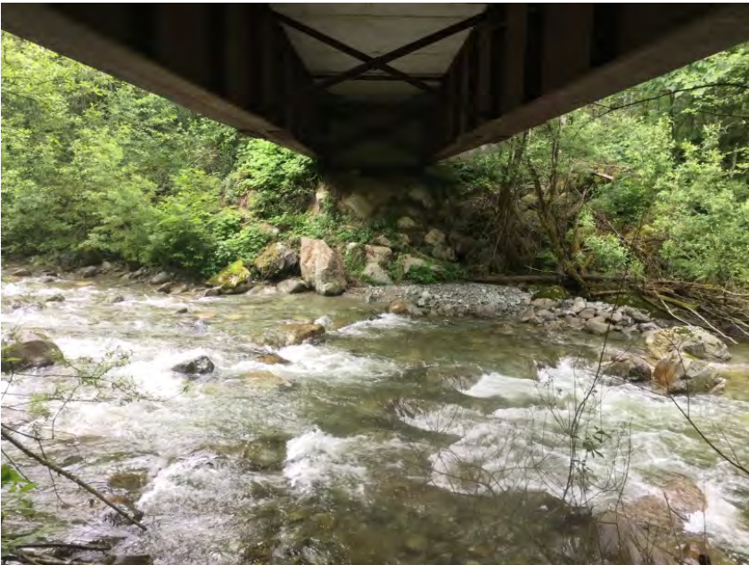
Left Bank Abutment when facing downstream
