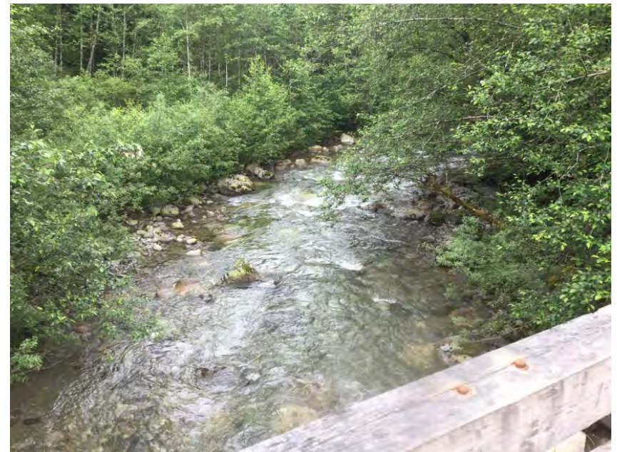
Looking downstream from deck
